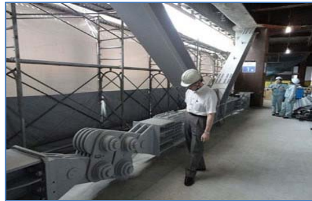
Fig. 10: Friction dampers
